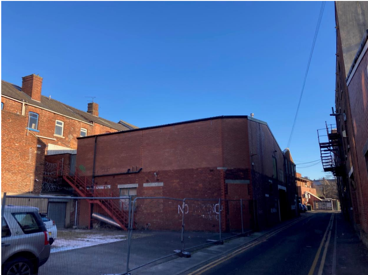
Photo 3: Existing building and two storey outrigger, viewed from Fleet Street
